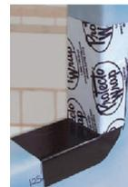
Cut Sill Tape 200mm long and apply to bottom of jamb and fold onto face of opening.
