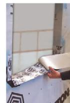
Cut Sill Tape to length, apply to sill and fold onto face of opening.
