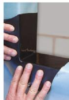
Peel plastic film from surface of Detail Tape and fold onto face of opening.
