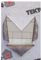
Cut wall underlay and staple to inside of opening.
