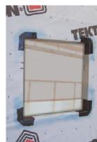
Detail Tape is required on all four corners of the opening. Press firmly into corners.
