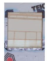
All tapes to be pressed firmly into place to maximise adhesion.
