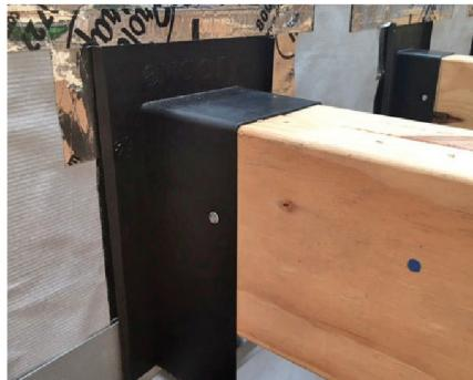
Tape sides and top of Pro-Joist back to underlay. Pro-Joist overhangs joist by minimum of 35mm.
