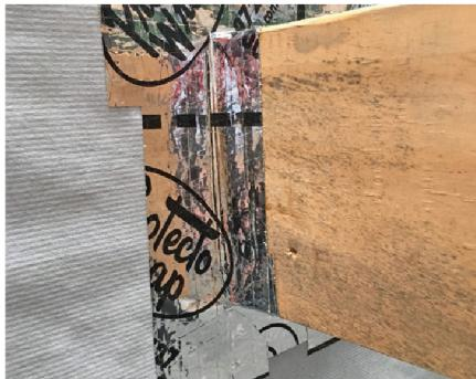
Building wrap taped around joist penetration back to underlay.
