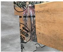
Building wrap taped around joist penetration back to underlay.
