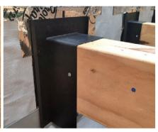
Tape sides and top of Pro-Joist back to underlay. Pro-Joist
