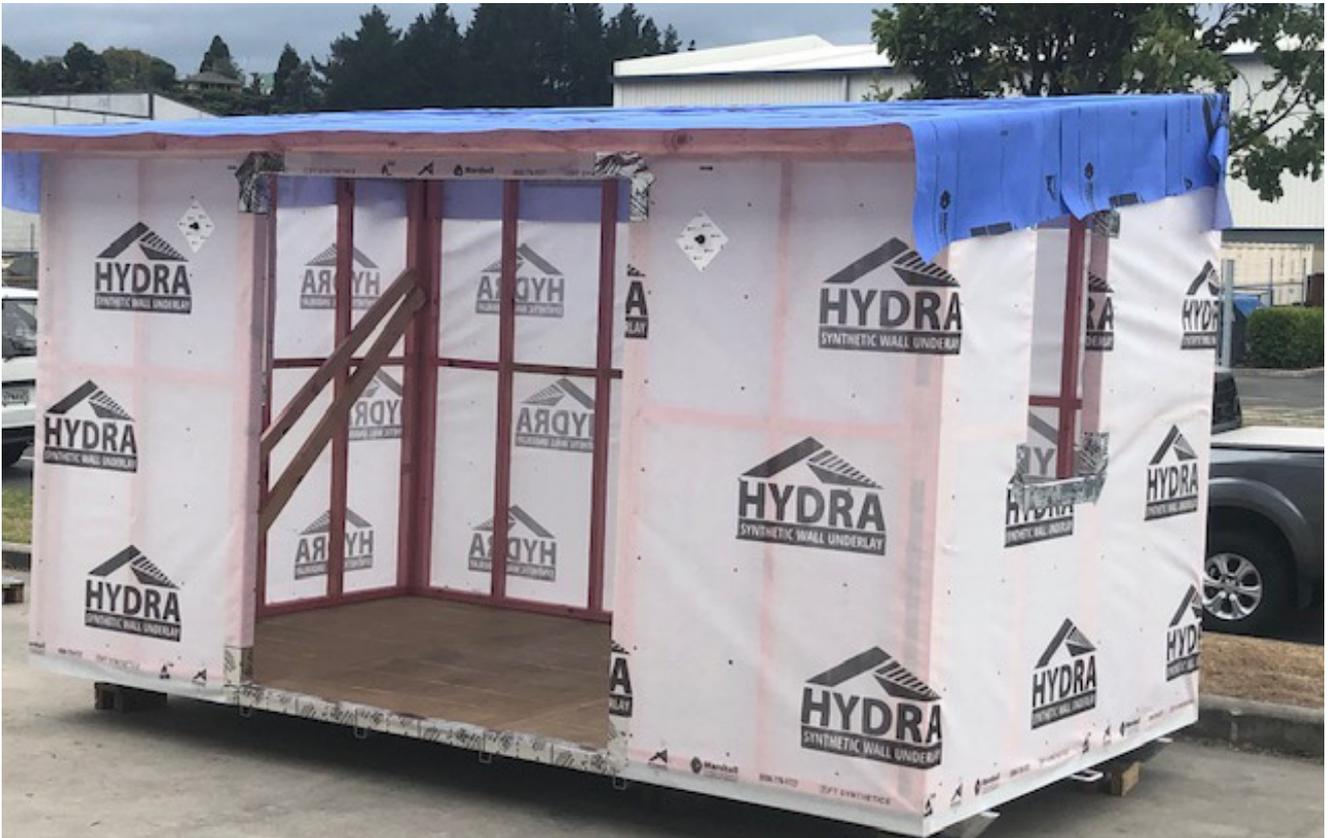
HYDRA Wall Underlay is an absorbent, breathable, fire retardant, flexible wall underlay used behind all wall claddings. Suitable with absorbent and non-absorbent claddings in both direct and non-direct fixing.
